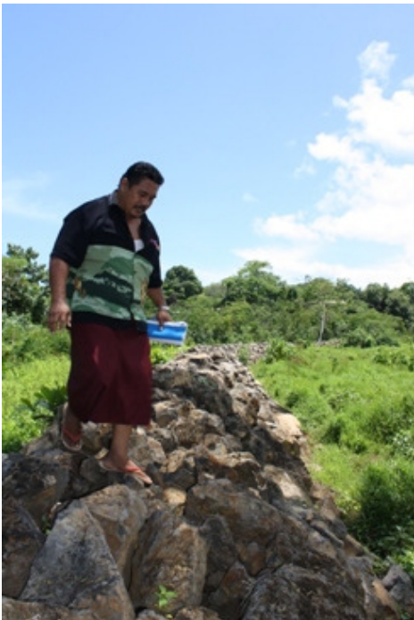
Figure 3: Tiuli Vao Foti, Salei'a CBA village committee member and a self-employed electrician, standing on the project site where a 200-metre retention wall was built and more than 200 trees were replanted along the stream against flooding and coastal erosion.
